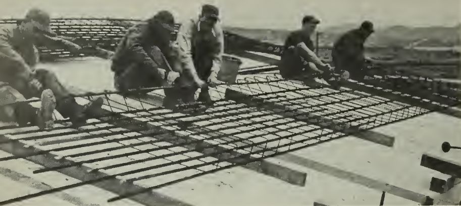
STEELING THE SHOW —Steel Workers assemble reinforcement for concrete.
